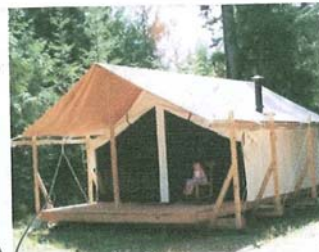
An example which shows how wood & fabric can be combined to form a practical shelter.
