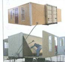
Very simple construction, panels simply fold out from a container.
