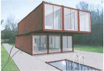
Portable shipping containers which are stacked together and form an interesting house.
